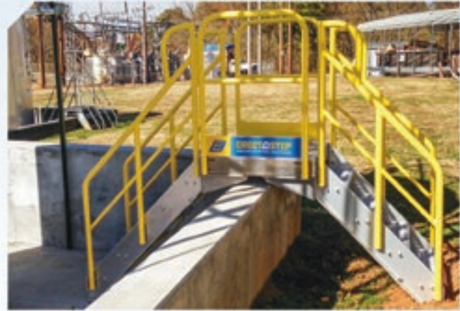
Safely cross containment walls.
