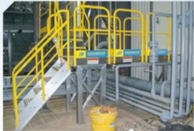
Multi-level access with inspection platform.
